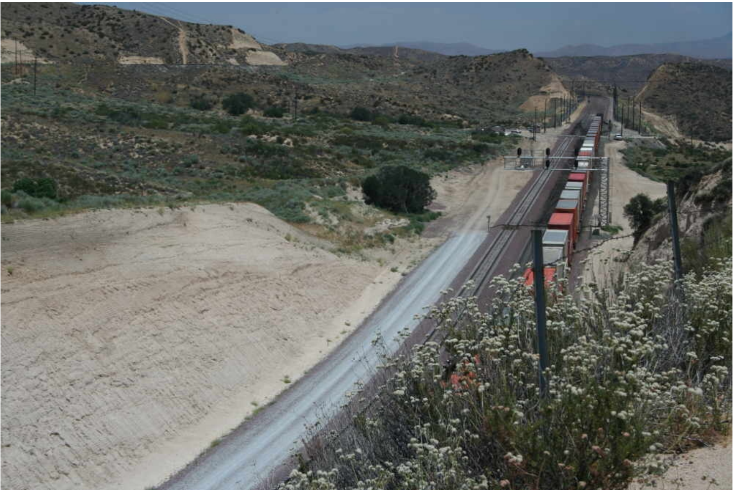
Photo on previous page shows a 100 car container train climbing up the grade to the summit. This page shows the train passing through the summit, headed east. The new third track is the one with the lighter colored concrete ties. Photos by Gerald Abegg.
