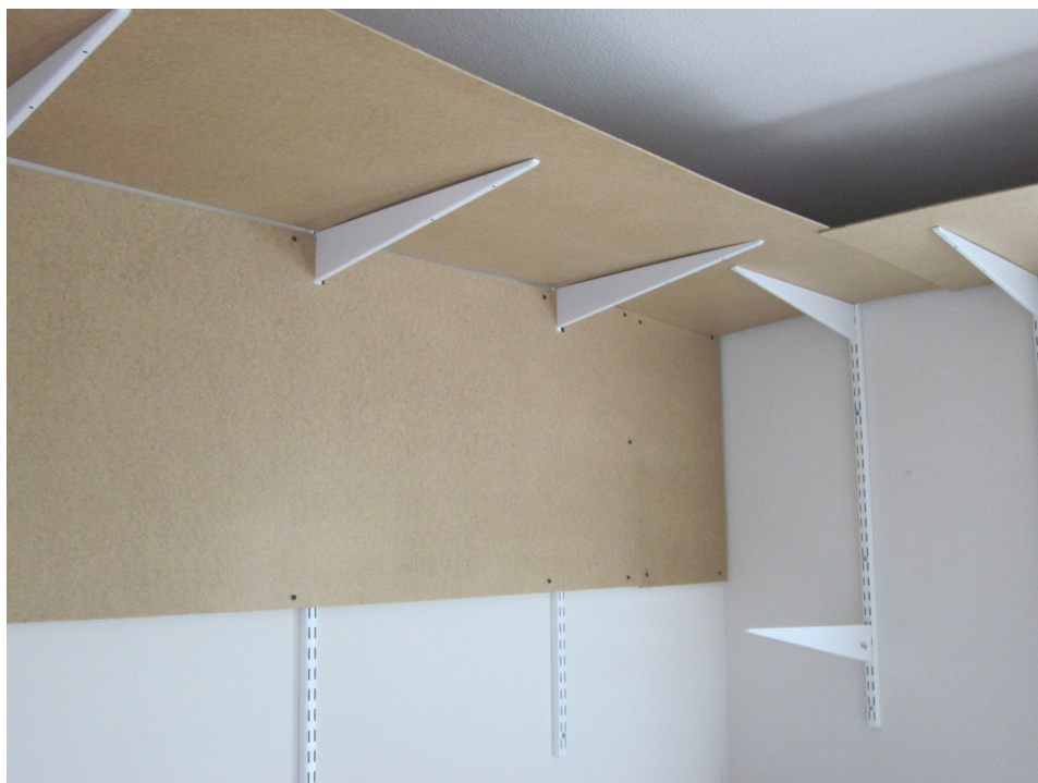
One corner under construction, showing shelving supports, hardboard backdrop and lighting
